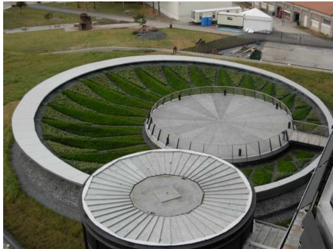
Green Roof, México (Green Roof Systems de México S.A.)
